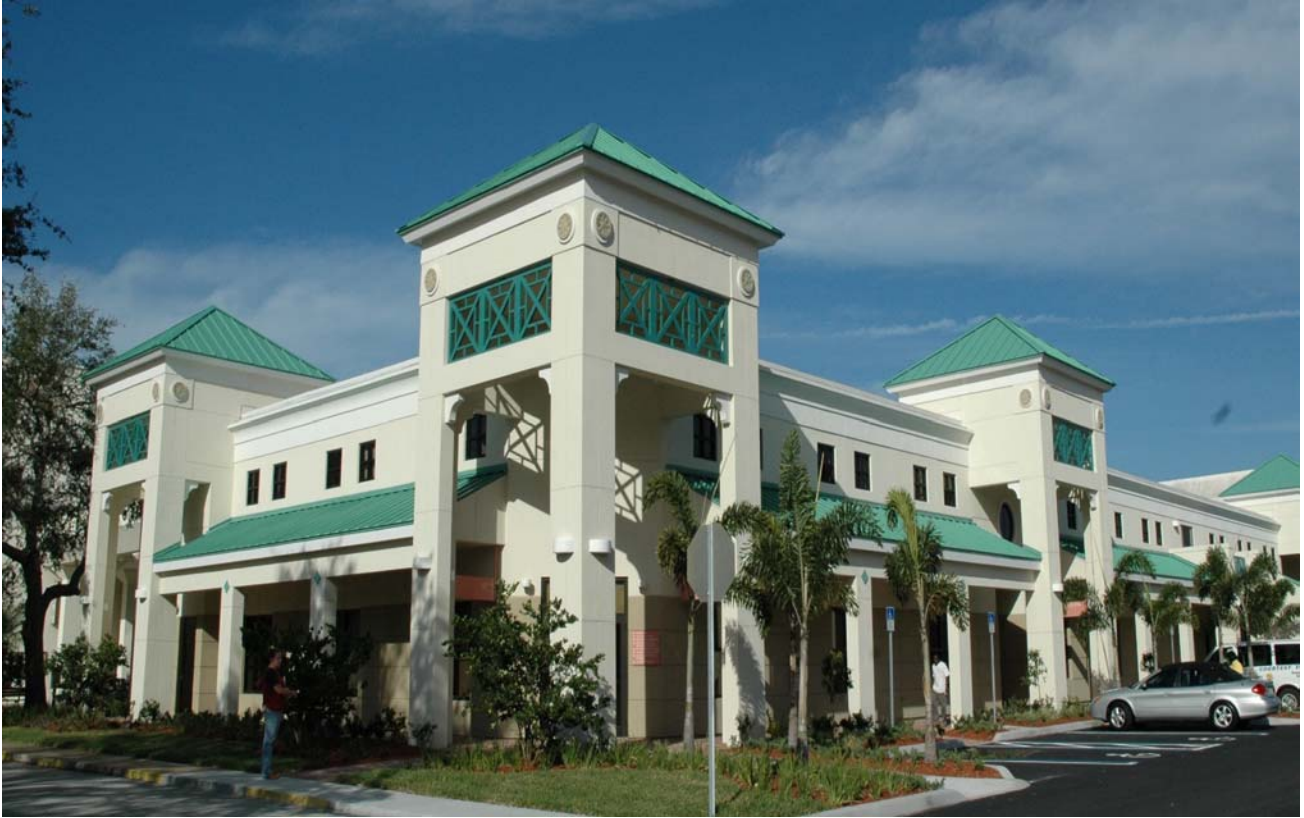
The New St. Lucie County Administration Building Addition on Virginia Avenue in Fort Pierce.
